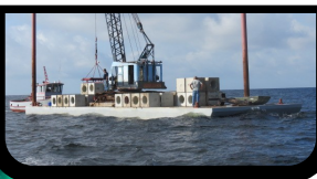
Deployment of Constructed Concrete Cubes.
