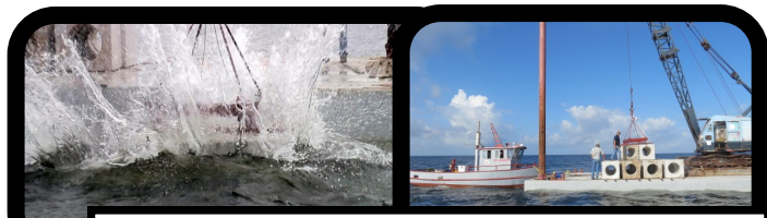
Deployment of Constructed Concrete Cubes.
