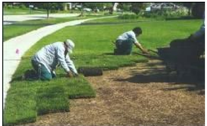
Figure 1. Sodding produces an instant lawn.
