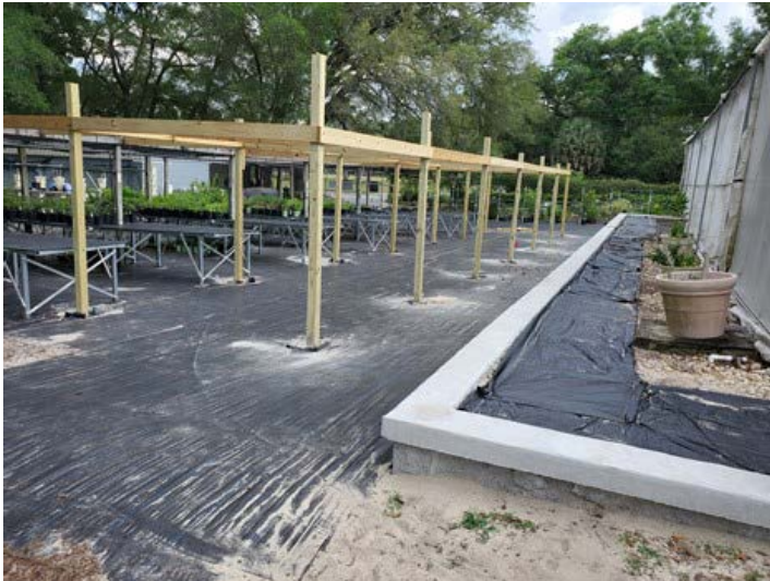
Construction on Marion County Master Gardener greenhouse retaining wall and benches.
